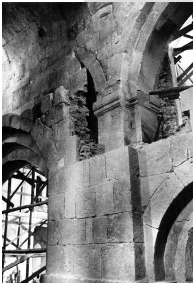
153. Svetitskhoveli Cathedral, wall opening process in 1970s
