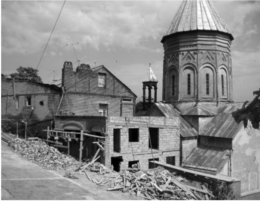
112. The loss of authenticity the use of non-traditional material (blocks) False restoration Tbilisi, Tsikhisubani 2010 photos
